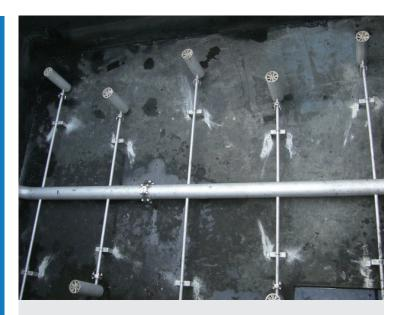
Wastewater type: Bus storage yard wastewaterVolume: 40m²/dayModel: Aquablaster system AL-750
