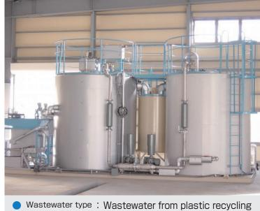
processes : 6~10m<sup>2</sup>/day Volume : Unit tank + AL-750 Model electrocoagulation flotation system
