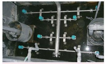
Circulating water type : Circulating water for painting Water tank : 30m<sup>3</sup>
