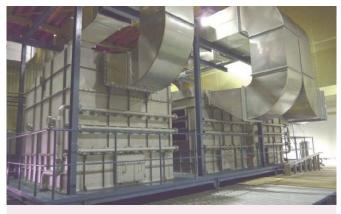
Circulating water type : Paint drying oven exhaust gas Water tank : 1050m<sup>2</sup>/min
