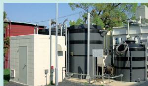
■ Shimadzu Corporation 10m 3 /day Kitchen wastewater treatment facility Cleaning water containing mineral oil is treated simultaneously
