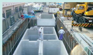
■ Kawasaki Food Industry Co., Ltd. Scene of wastewater treatment facility construction Seven 40m 3 unit tanks
