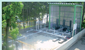
■ Kyokuto Kaihatsu Kogyo Co., Ltd. 50m 3 /day Mineral oil effluent treatment facility Release of highly concentrated mineral oil is also stopped
